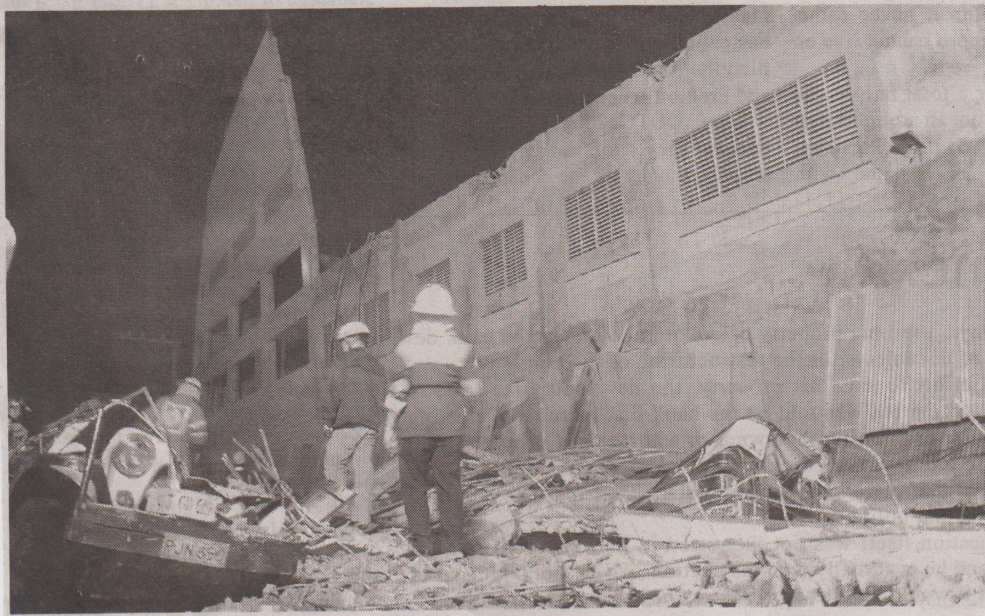
Rescuers look for survivors after a building wall collapsed on May 19, 2014 in Masambong, Quezon City. DANNY PATA
